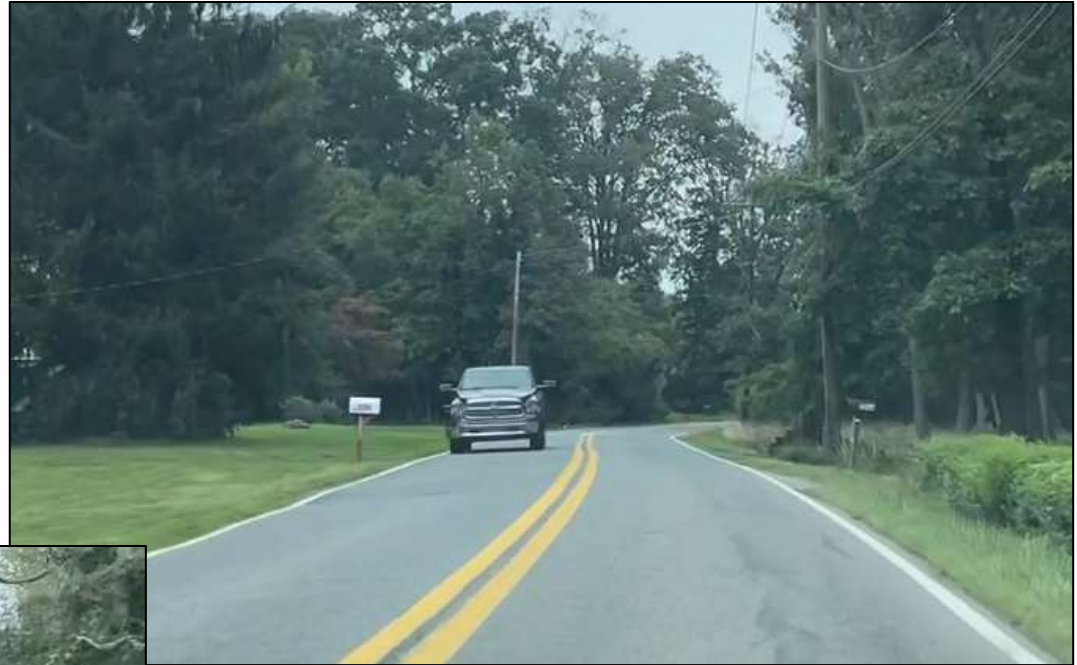
Old County Road Eastbound Approach
