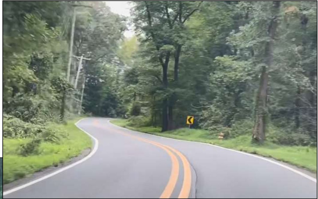
Old County Road Eastbound Approach
